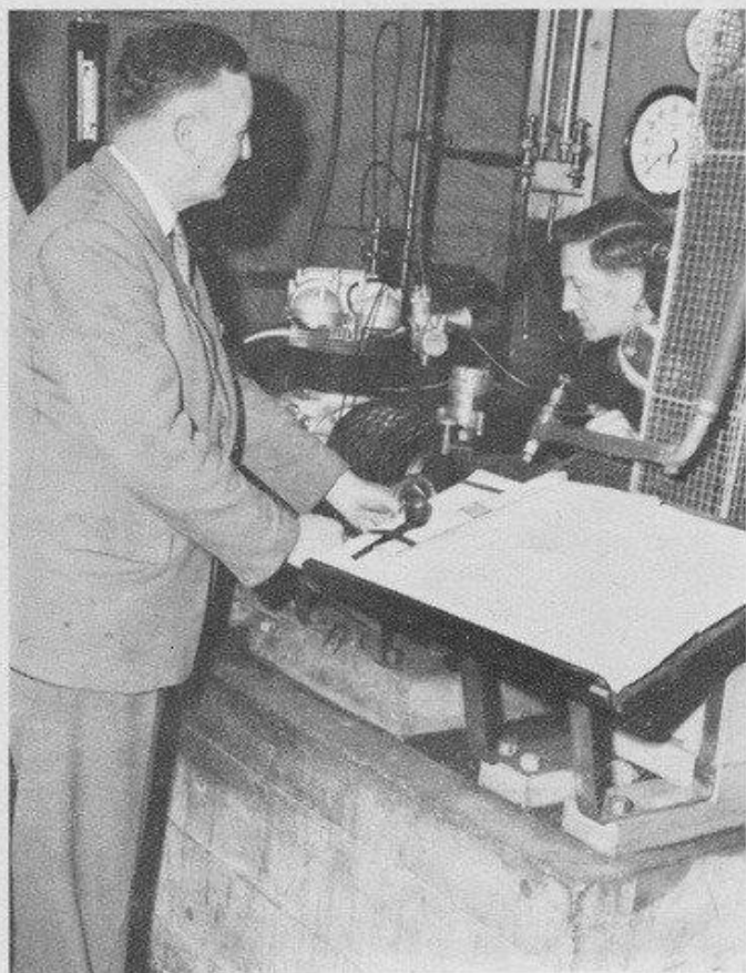
Development engineer Jack Williams and his assistant, Fred Wynn tests a new engine in the small underground engine testing room. The resistant load against which the engine is pitted, is supplied by water pressure against vanes fitted on the driving side of the engine crankshaft
