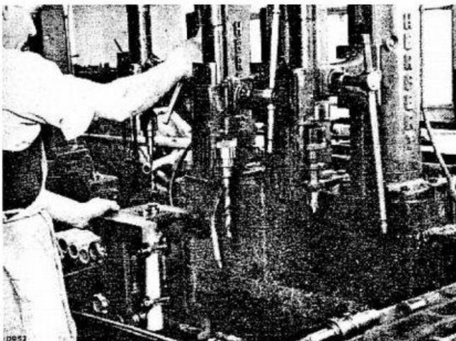
In addition, the entire slider is brought to a  $1 \frac{9}{16}$ " diameter over a length of more than 10". The slider is first pre-rotated, then accurately turned and then the reamer goes through. In these three operations, the turret remains in the same position and the tool must therefore be able to be changed quickly. A laborious stage and the entire cycle takes no less than 11 minutes.
